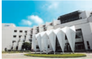
Tainan Plant (Diamond-rated Green Building)
