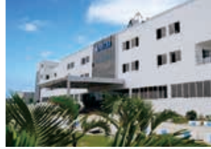
Rudrapur Plant (Green Building)
