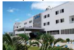
Rudrapur Plant (Green Building)
