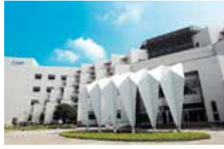
Tainan Plant (Diamond-rated Green Building)
